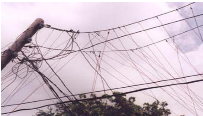
Figure 1.0 – An example of a ‘throw-up’ – a common form of electricity theft.
